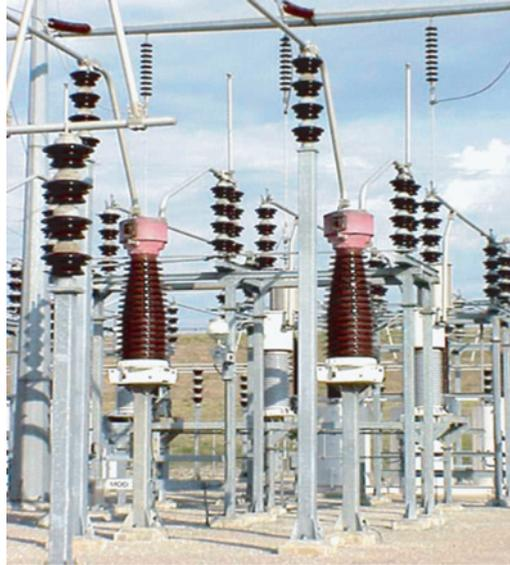
Conductors and insulators. Copper, aluminum and silver (if you can afford it) make good conductors. Pyrex, porcelain and ceramics like alumina make good insulators – they are dielectrics. (Images courtesy of the Copper Development Association.)
